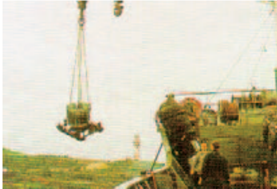
Transfer of an RTG onto a ship for further transport (Photo: Office of the County Governor of Finnmark).
