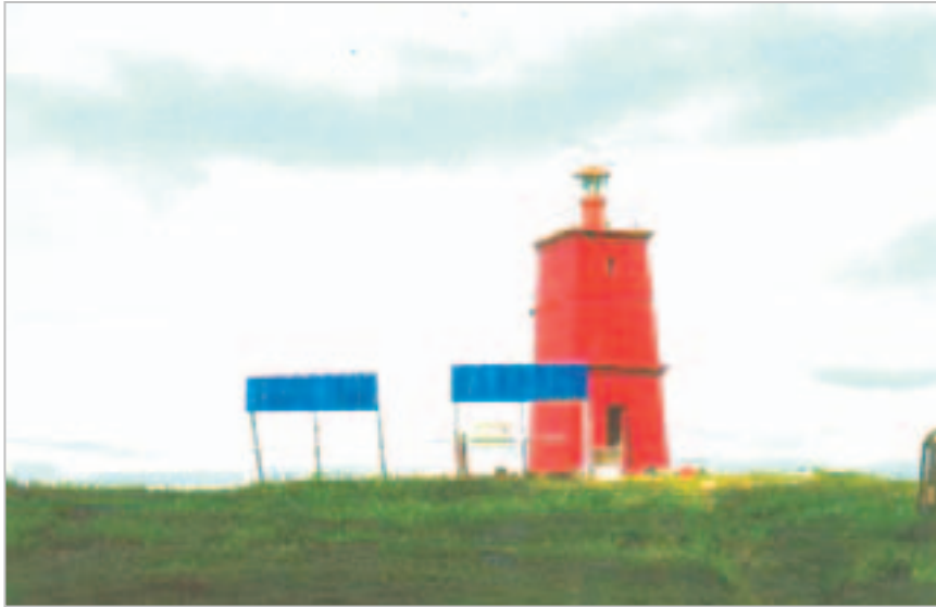
A new lighthouse running off solar power
