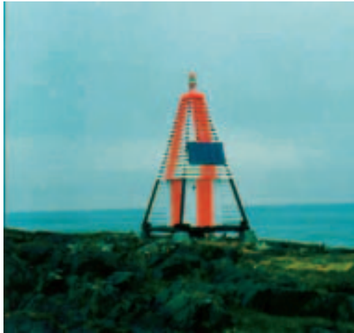
An alternative to RTGs: A lighthouse fitted with a solar panel that generates electricity (Photo: Office of the County Governor of Finnmark)
