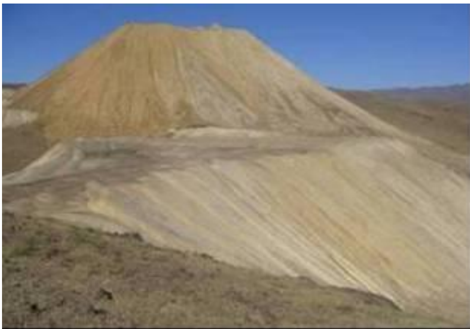
Fig. 5. Waste of dumps of the “poor ores mill” formed until 1965. It is one of the facilities requiring rehabilitation.
