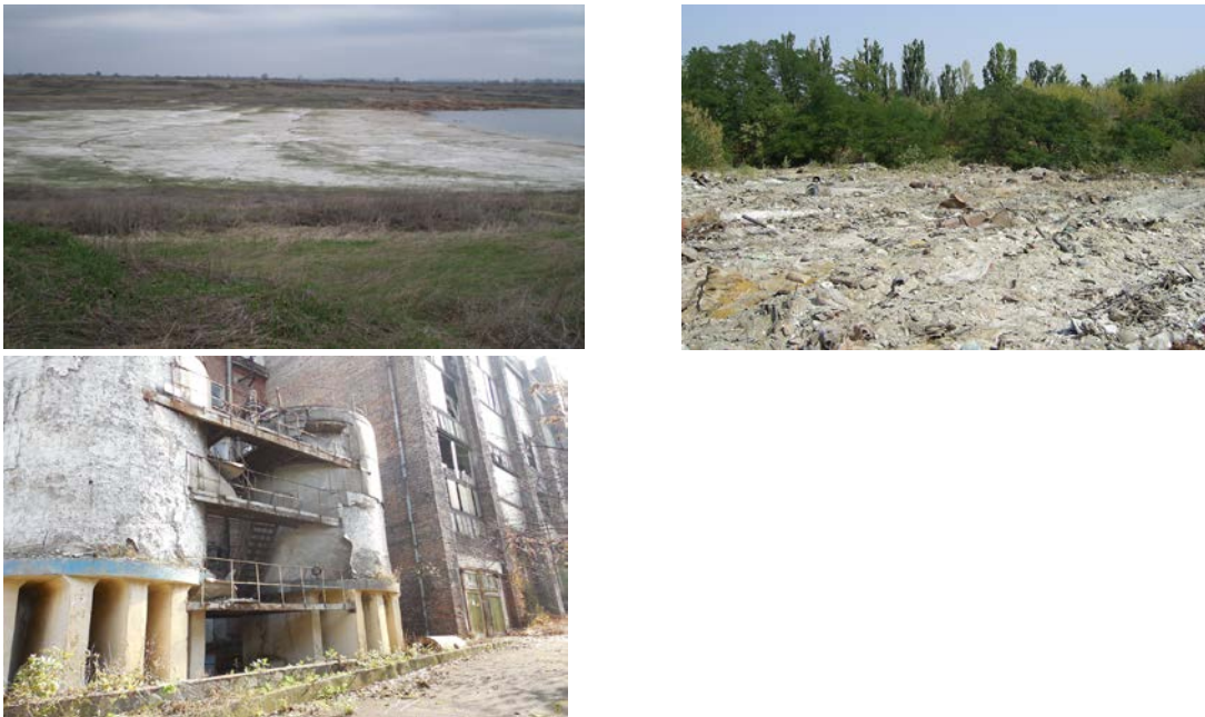
Figure 25. Pridneprovsky chemical plant tailings ponds and technological sumps building. Upper left – tailing pond Sukhachevskoye, upper right – tailing pond Yugo-Vostochnoe, lower – Building 103 Technological sumps.
