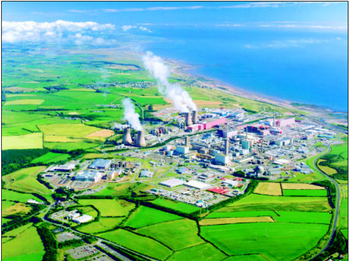
Figur 6: Sellafieldanlegget (foto: BNFL).
