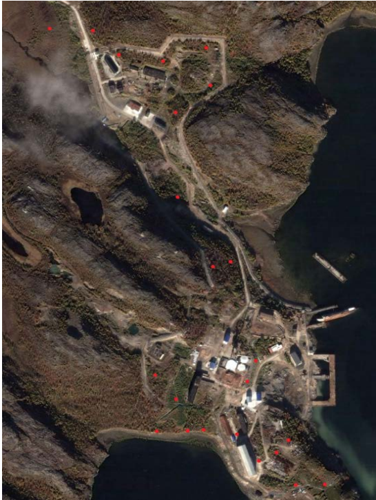
Fig. 8A Points for the soil sampling on the industrial site
