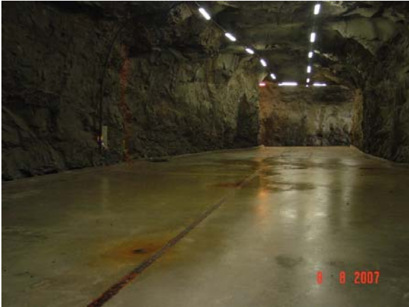
Figure 4. Photo of the largest repository tunnel.
