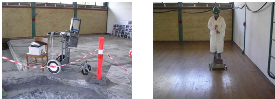
Figure 1. Clearance measurements performed inside the DR 1 reactor hall. The left-hand picture shows \gamma -spectrometric measurements of the “crater” and the right-hand picture shows contamination measurements of the floor with an \alpha -/ \beta -contamination monitor.
