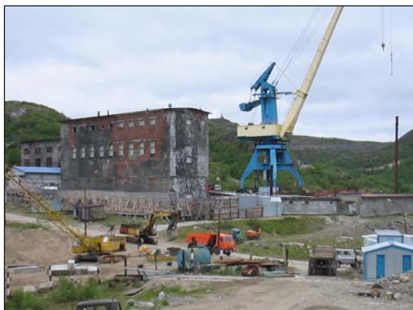
Overview of Building nr. 5 at Andreyev Bay.
