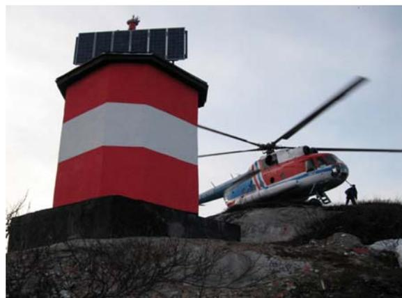
*A RTG lighthouse in Northwest Russia replaced with solar panel (Photo: The County Governor of Finnmark).*
