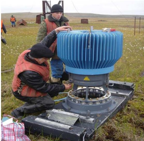
Removal of a RTG from its original placement in Northwest Russia (Photo: County Governor of Finnmark).
