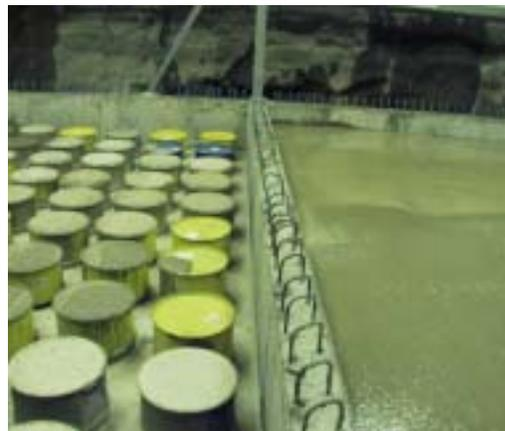
*Embedding drums and containers in concrete in section 3 and 4 of hall no. 4.*
