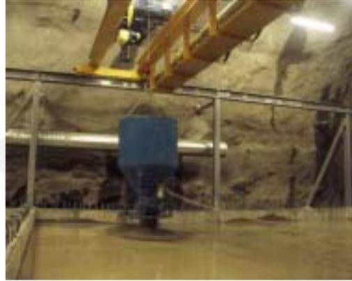
*Embedding waste packages in concrete in section 4, hall no. 4.*
