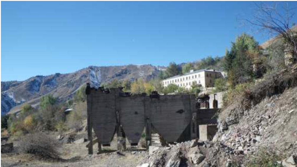
Fig. 10. Former ore concentrating plant in Yangiabad
