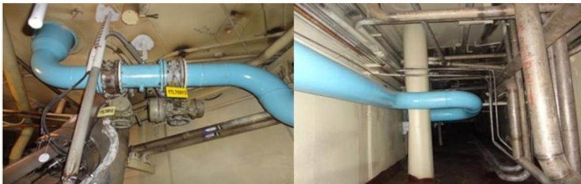
Fig. 3.3 Implementation of the filtered containment venting concept in the event of a severe accident at SUNPP-1
