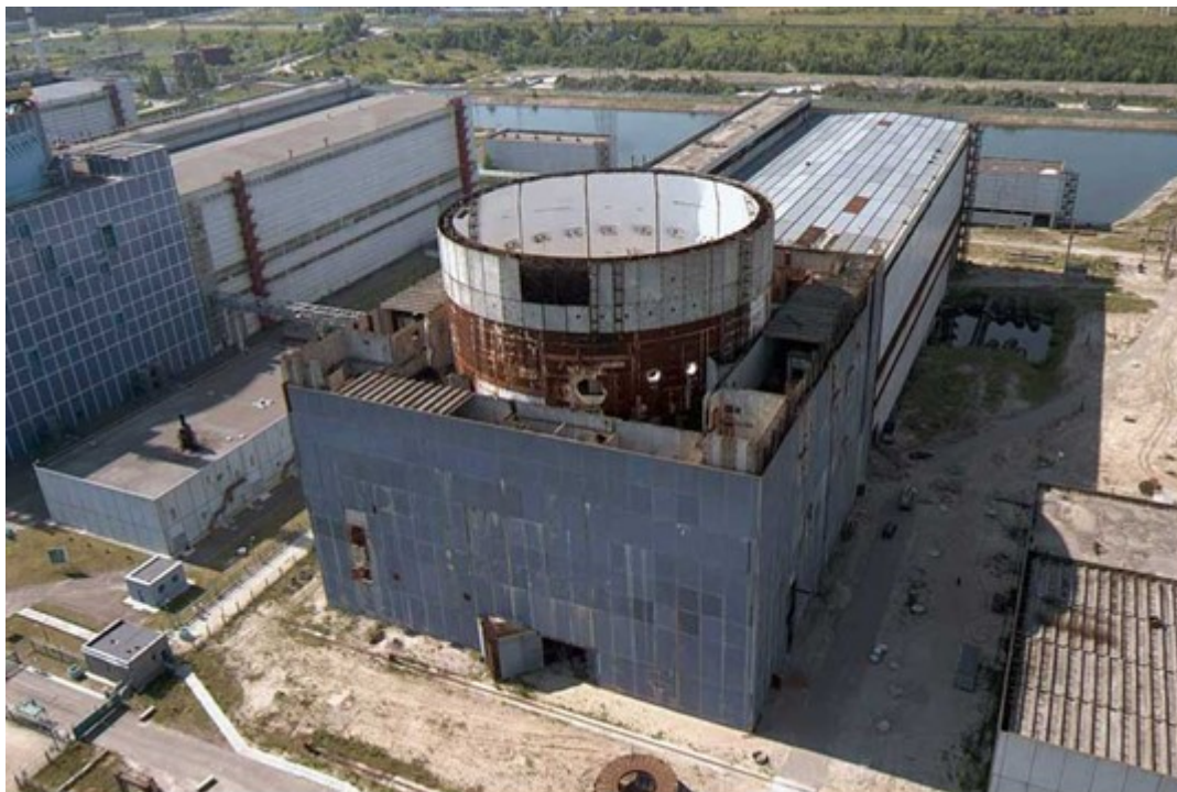
Figure 2.5 – Khmelnytsky NPP unit 3
