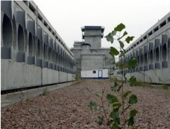
Figure 5.7 – ChNPP dry interim spent fuel storage facility
