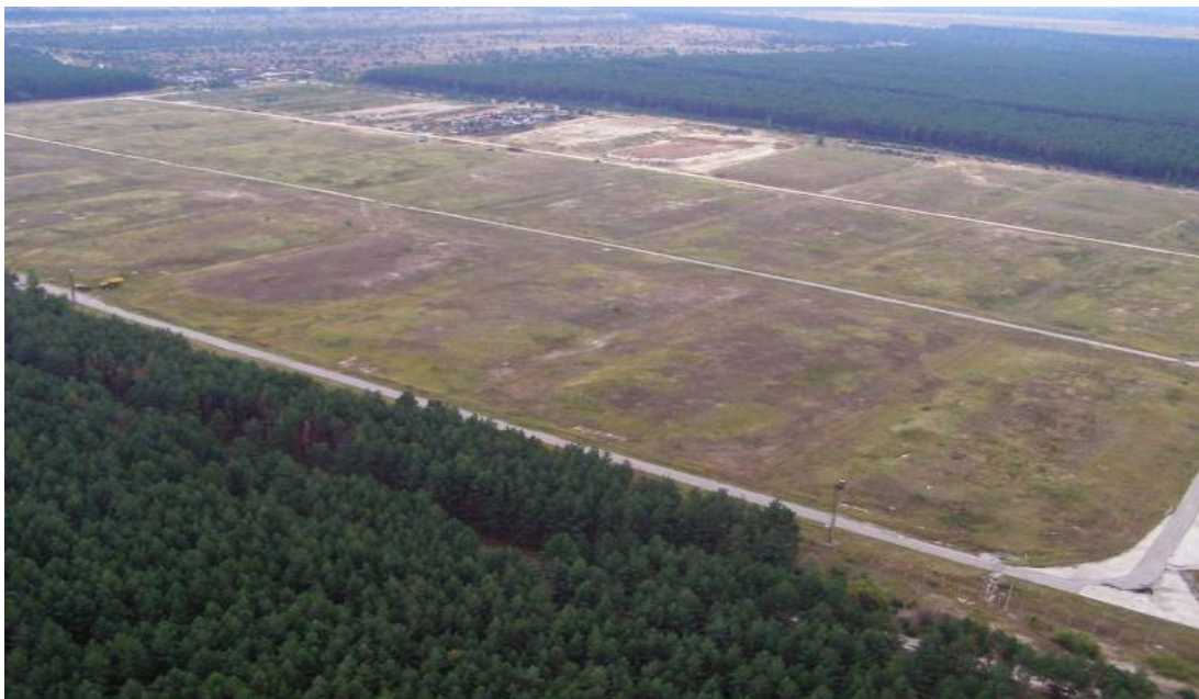
Figure 5.2 – Buryakivka disposal facility for short-lived Chernobyl-origin radioactive waste
