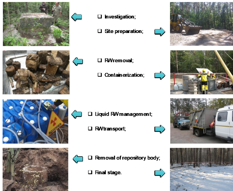
Figure 10: Stages in the remediation of the military radioactive waste storage site Vakulenchuk.
