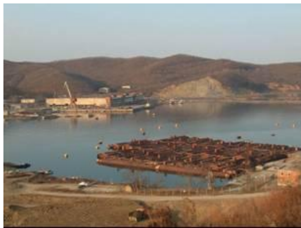
Fig. 2.6.2. Three-compartment reactor sections from dismantled NPS in a floating temporary storage facility at Razboynik Bay
