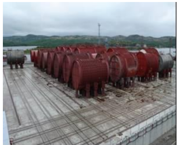
Fig.2.6.8 Disposition of reactor compartments in a long-term storage stations at "Saida" LSF
