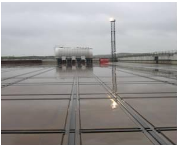
Fig. 2.6.7 Reactor compartment in a long-term storage station at "Saida" LSF
