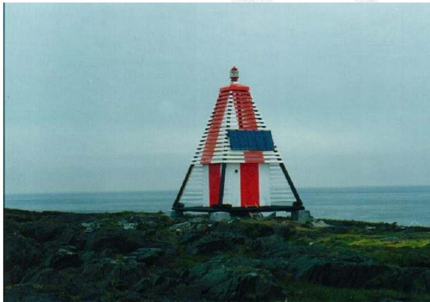
*An alternative to RTGs: A lighthouse fitted with a solar panel that generates electricity.
