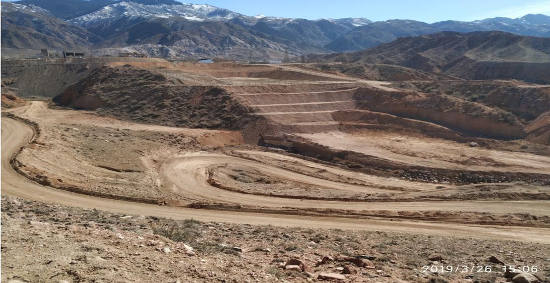
Figure 10. Completion of the remediation at Kaji-Sai tailing pond (strengthening of the slopes of the storage, construction of a new dam, construction of a mudflow allotment, surface restoration), March 2019
